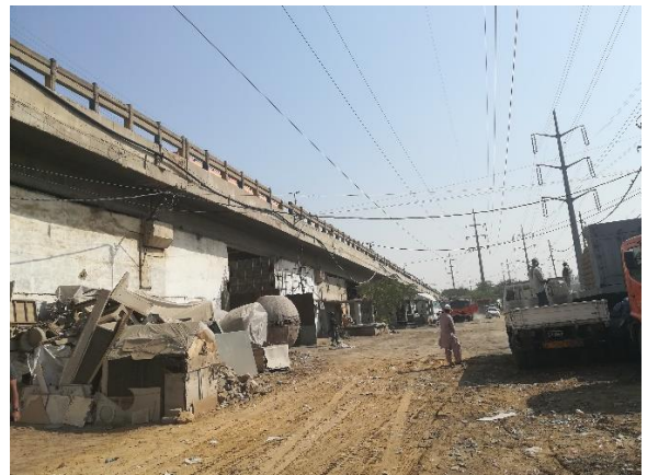
A view of Stores Under Bridge
