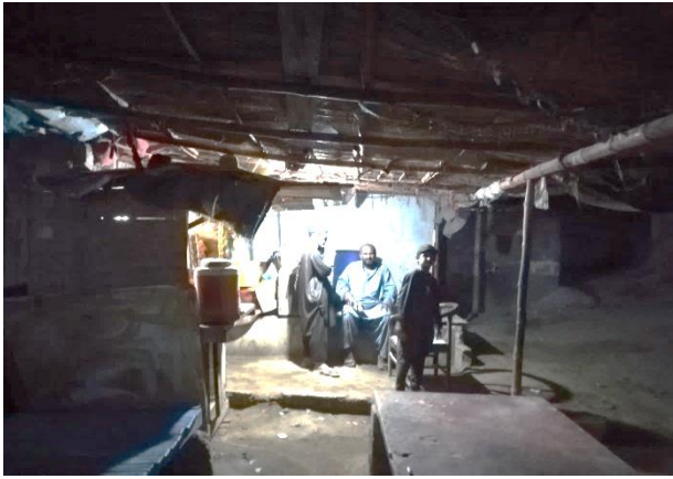
A view of Temporary Tea Stall Under Impact
