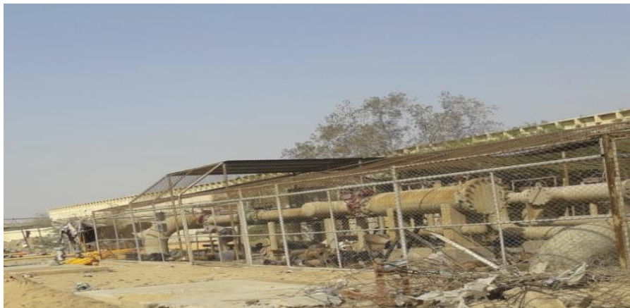
Figure 3-1: Gas Station at Jam Sadiq Bridge Under impact
